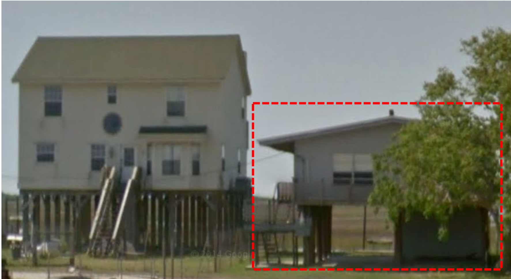
Before Harvey hurricane in Rockport, TX (Google Street View)
