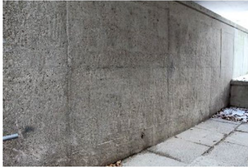
Building Wall (BW)
