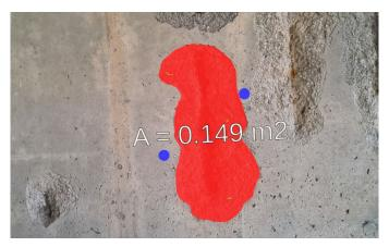
• Step 4: Calculate area of final segmented damage region
