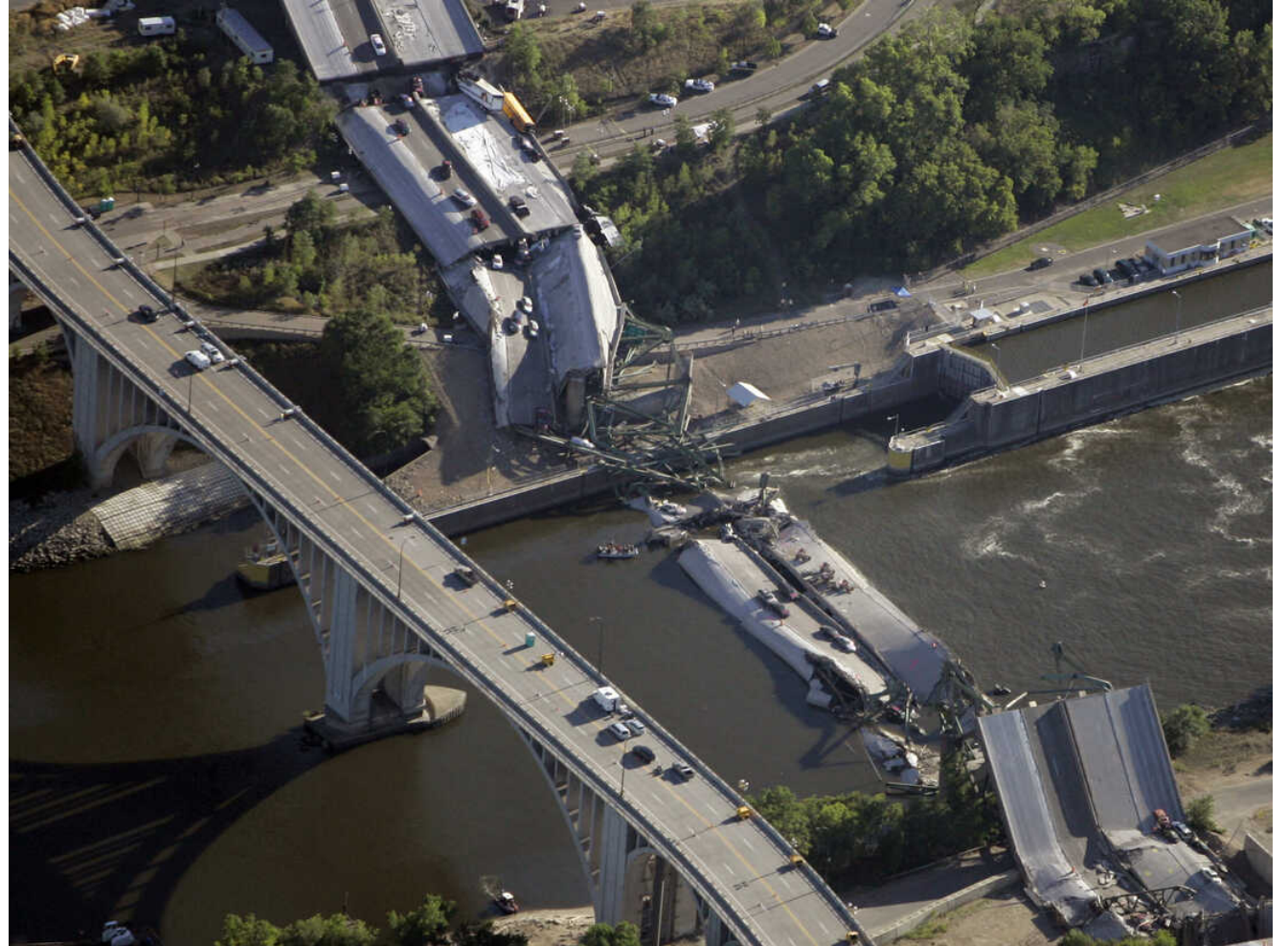
I-35W Mississippi River bridge collapse ( source: NPR )
