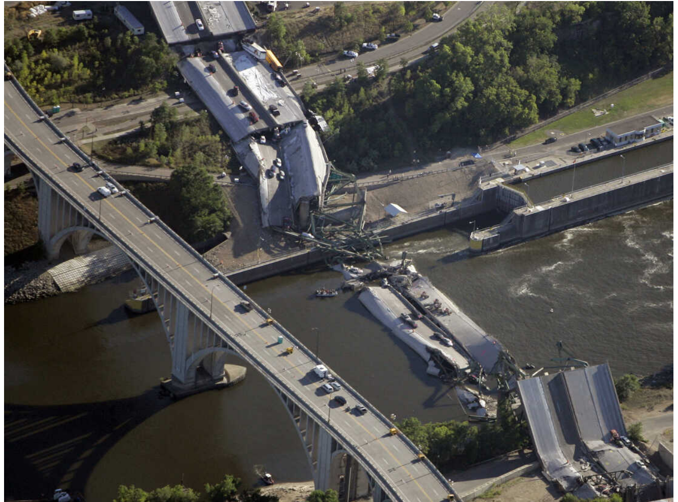
I-35W Mississippi River bridge collapse ( source: NPR )
